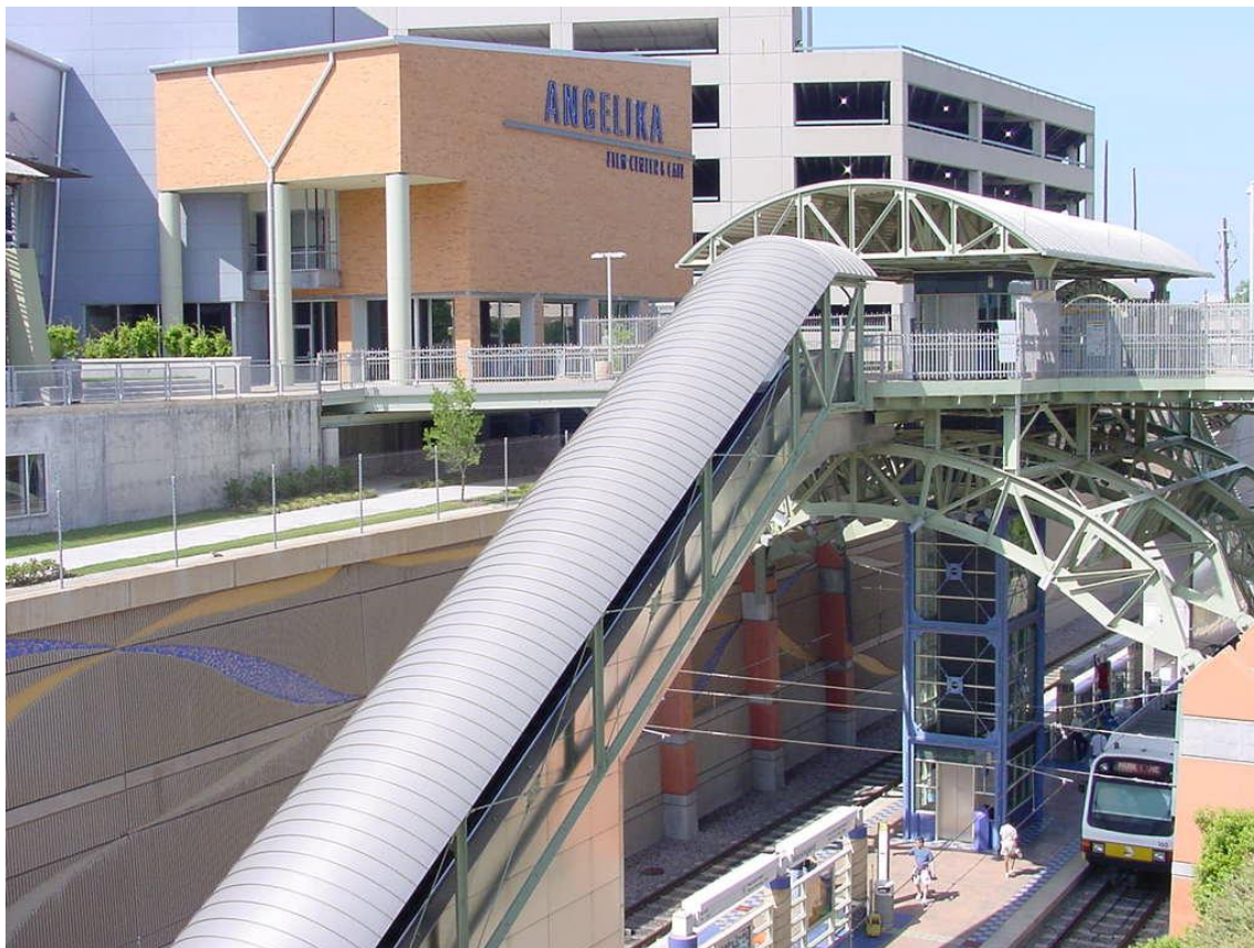
Figure 2: DART Mockingbird station, Dallas TX
