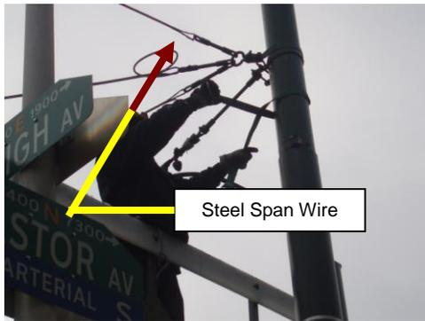
Figure 2. Trolley Wire Support with Steel Span Wire
