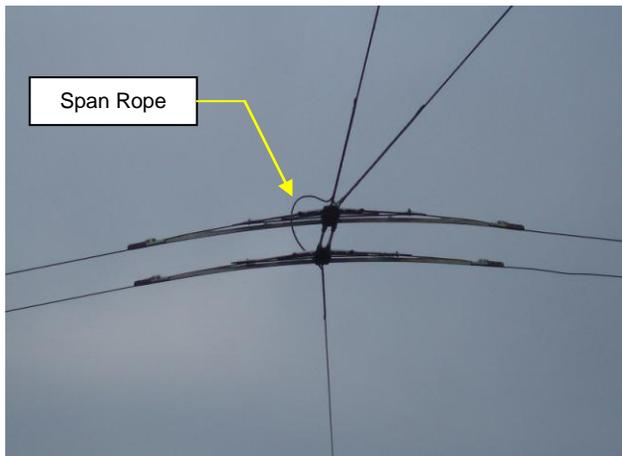
**Figure 5. Span Rope Connecting Trolley Bus Wires**
