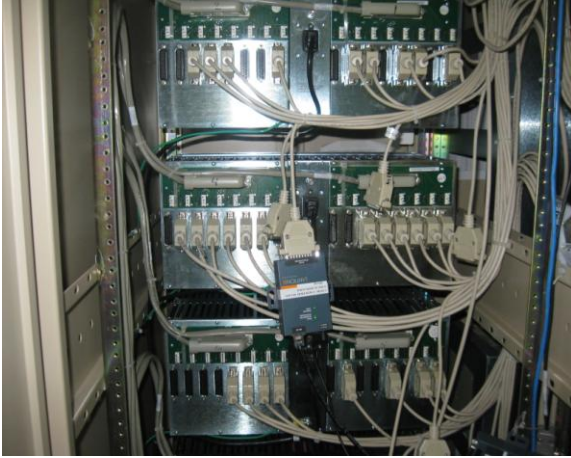
Figure 7 UDS 1100 connected into network
