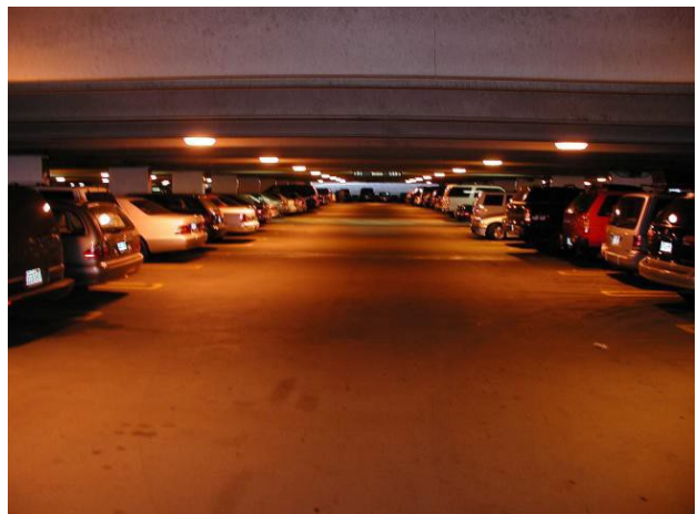
High-pressure sodium installation Correlated color temperature: 1900 °K Color rendering index: 22
