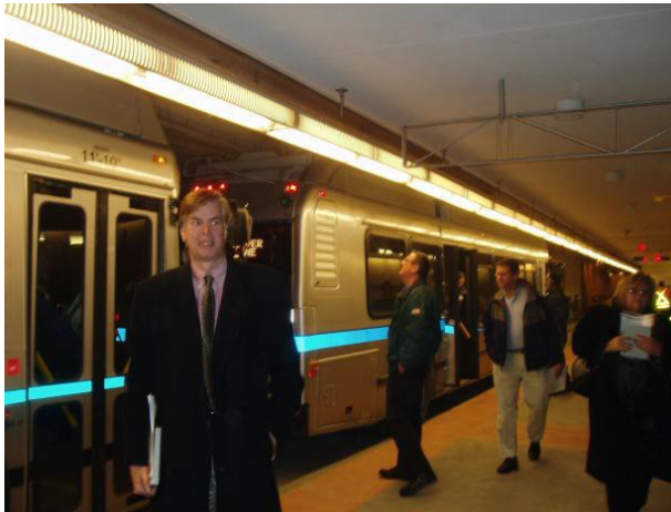
FIGURE 4 Platform Edge Lighting
