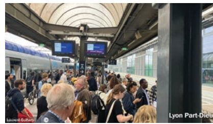
Figure 9 - Lyon Part-Dieu opened in the early 1980s, expecting 35,000 daily passengers. Today, it serves over 140,000, four times that amount. The narrow platforms from decades ago still limit capacity. Crowding can lead to safety risks, as the photo shows.
