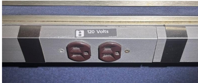
FIGURE 3 Surface-Mounted Raceway Installation
