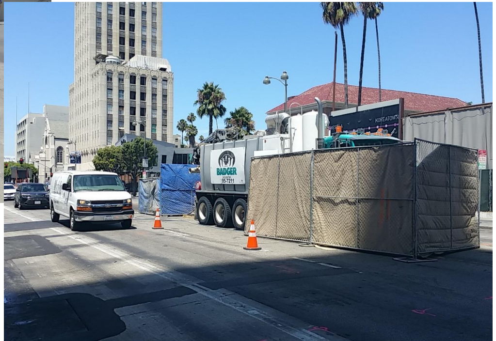
C1045 170727 1204pm STS Badger Potholing Behind Sound Barriers on Wilshire W of Western facing NW
