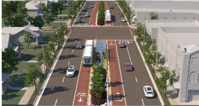
Median Busway with Center Station and Left Side Boardings
