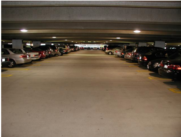
Metal halide installation Correlated color temperature: 3700 °K Color Rendition Index: 70
