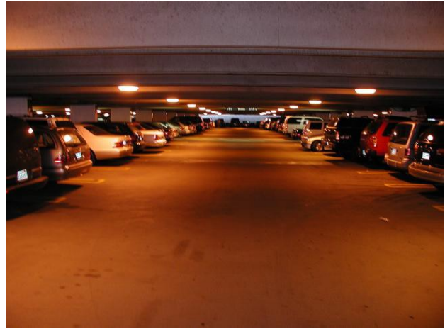
High-pressure sodium installation Correlated color temperature: 1900 °K Color Rendition Index: 22
