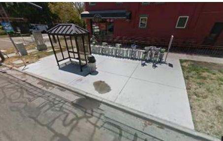
The Utah Transit Authority (UTA) has installed multiple bus stop pads with additional concrete area to accommodate future bike-share stations.
