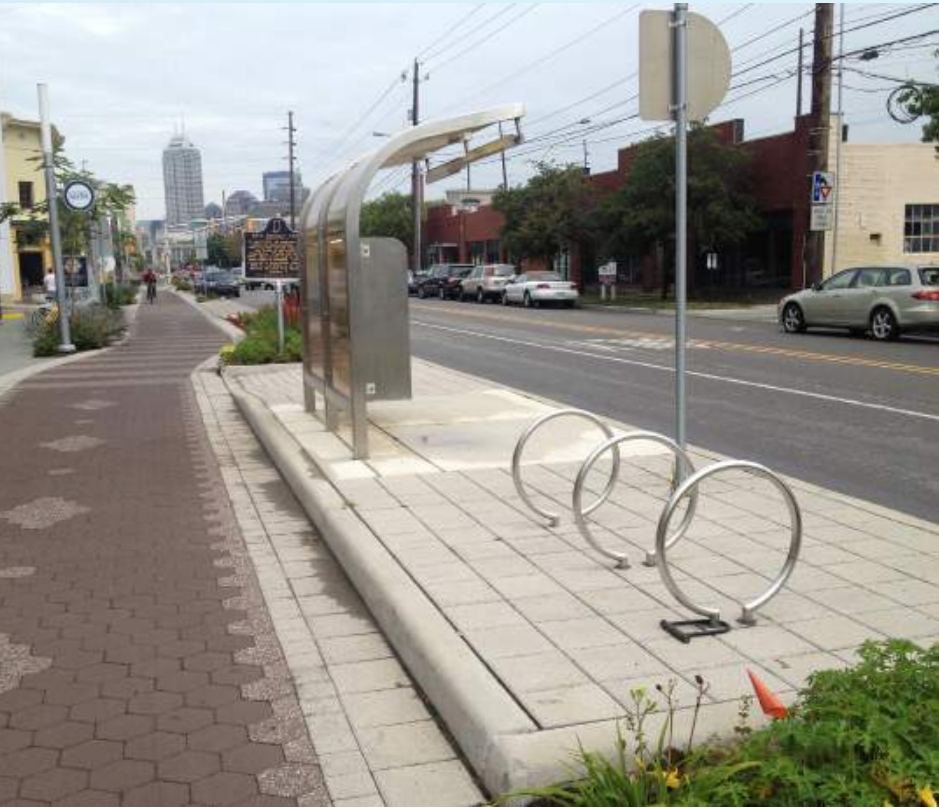
This design provides a physically separated bicycle ROW adjacent to an island bus stop and marked pedestrian crossing.(Cleveland, Ohio)
