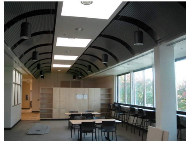
Ryerson Transit Base Interior Retrofit
