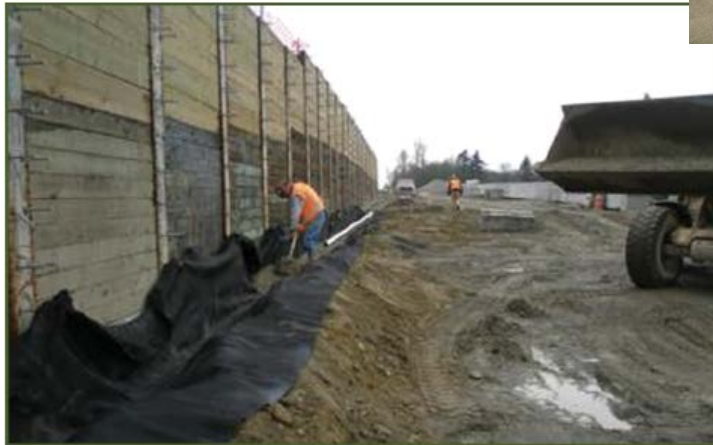
Bow Lake Recycling and Transfer Station
