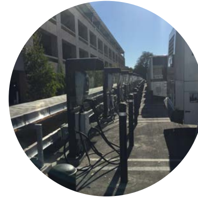
Charging and microgrid at facility
