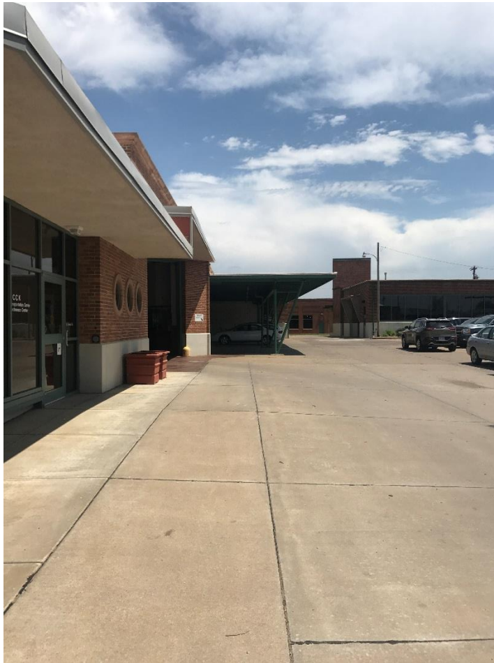
Figure 1: OCCK, Inc. Administrative and Maintenance Facility (Photo: TranSystems)
