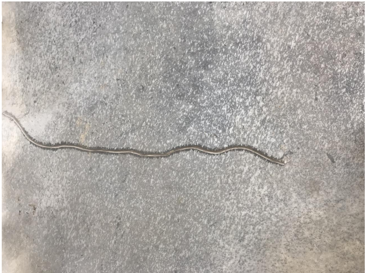
Figure 1: ATA Floor Cracking Repair Example (Maintenance Area) (Photo: Groundswell Consulting)
