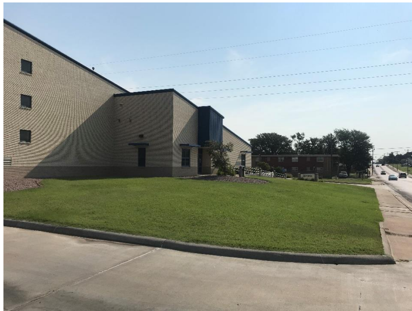
Figure 1: Access Transportation, DSNWK's Administration and Maintenance Facility (Photo: TranSystems)
