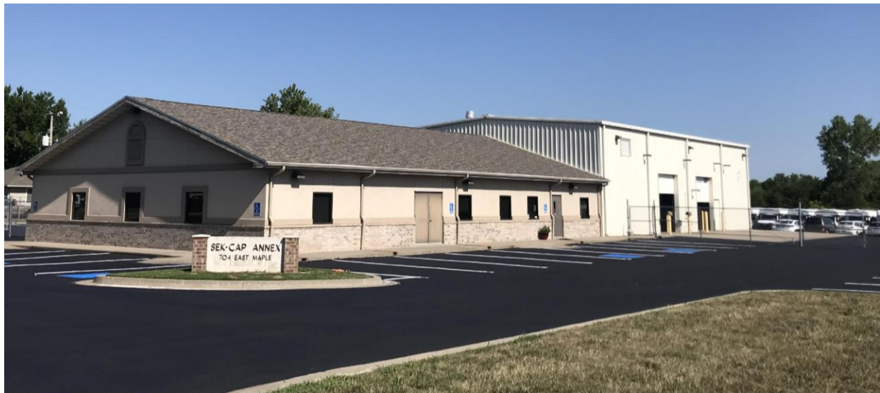
Figure 1: SEK-CAP Administrative and Maintenance Facility (Photo: Groundswell Consulting)
