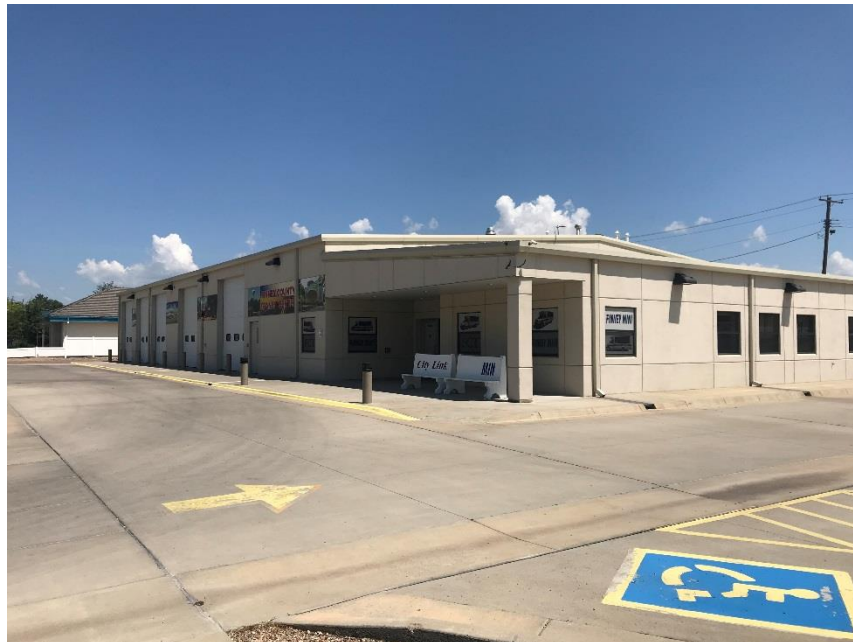
Figure 1: Finney County Administration and Maintenance Facility (Photo: TranSystems)
