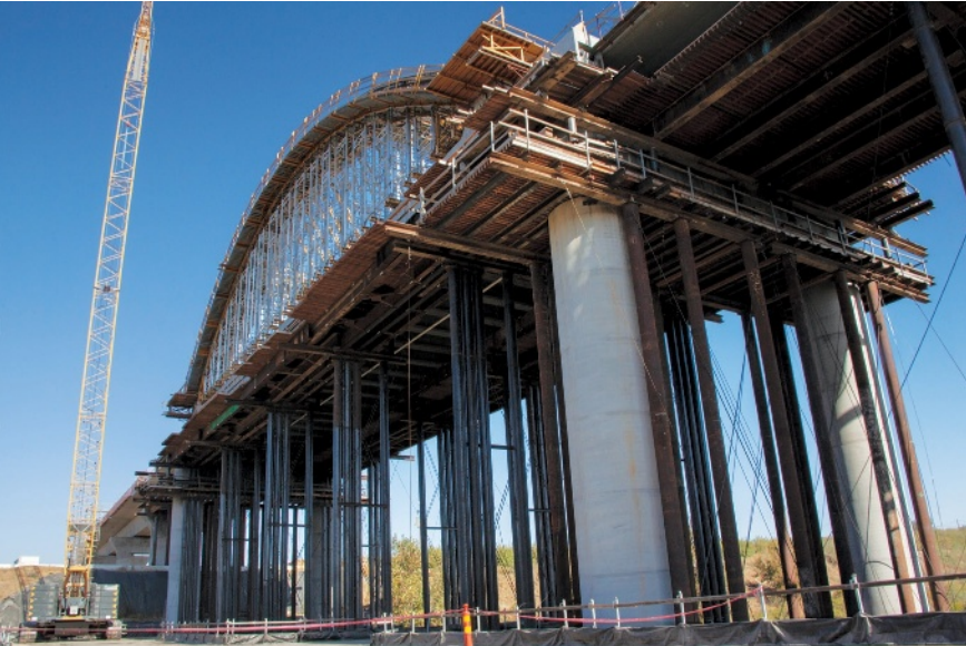
In north Fresno, crews are working over the San Joaquin River and making final preparations before placing concrete at the east archway of the viaduct (Nov. 2019).
