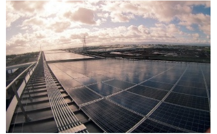
Solar panels throughout BART's Warm Springs Station provide enough energy to meet the station's daytime power needs.
