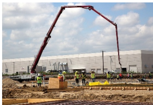
Workers pouring concrete at the TEXRail Equipment Maintenance Facility.
