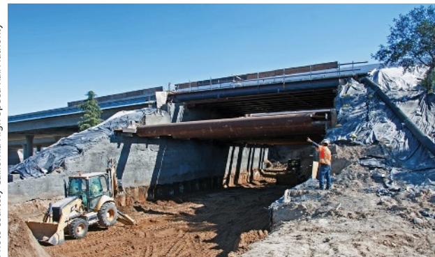
Construction on the Fresno Trench beneath State Route 180. A 10-foot-tall, three-foot-thick barrier wall will separate the high-speed rail alignment from the existing freight rail that parallels the project.
