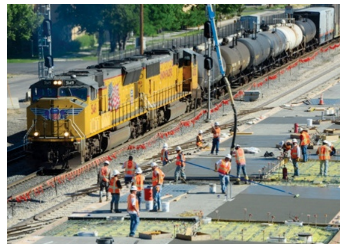
UTA contractors placing concrete for a FrontRunner commuter rail station platform in the rail corridor shared by Union Pacific.
