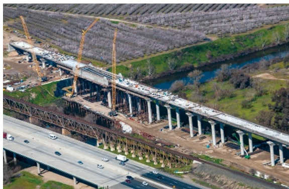
At the San Joaquin River, crews are seen installing metal decking over the river, concrete superstructure elements are being poured to the south of the river and deck drainage is being installed on completed sections.
