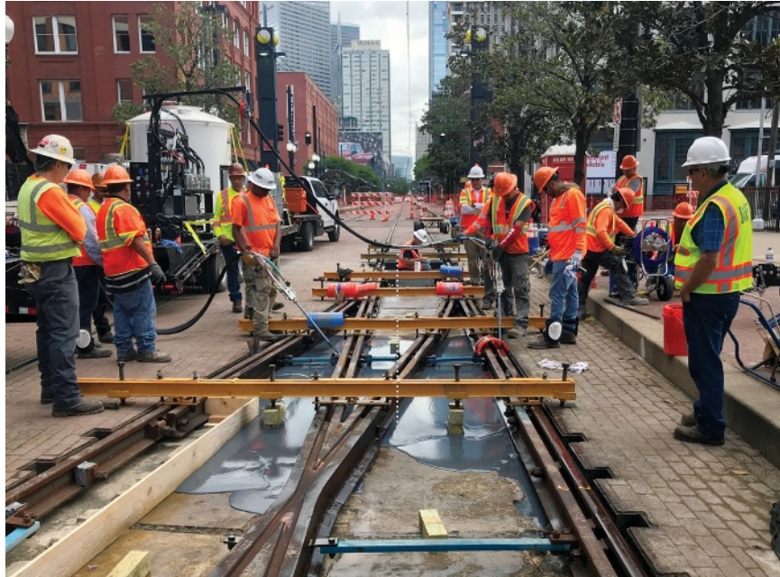
DART found that HPRE-MD provided superior noise and vibration reduction for its downtown Dallas business district rail replacement project.
