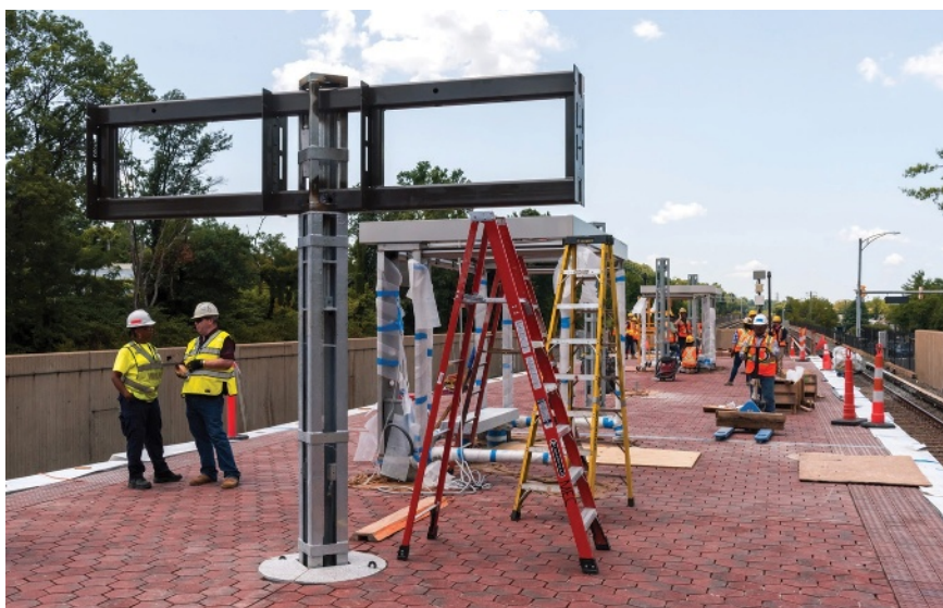
Metro took advantage of the shutdown to also improve the customer experience with the installation of new slip-resistant tiles, platform shelters with charging outlets/USB ports, larger digital next-train signs, energy-efficient LED lighting and clearer public address systems.
