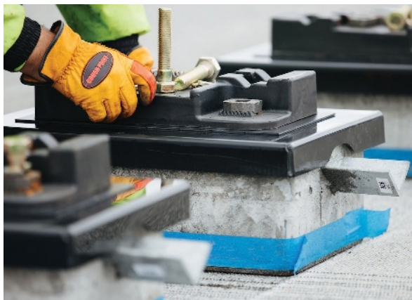
Specially designed and manufactured lightweight concrete blocks support the tracks on the I-90 bridge. The blocks are attached to the bridge deck using a high-strength epoxy. A drip cap on top of the blocks, and a layer of corkelast on the bottom, isolate stray current from the electrical system that powers the light rail vehicles and protects the bridge structure from corrosion.
