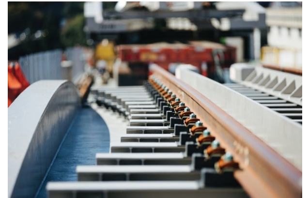
Engineers designed a structure called a track bridge to enable light rail vehicles to travel smoothly from land onto a moving, floating bridge. While it is a completely new solution, the track bridge is constructed with materials commonly used in seismic retrofits.
