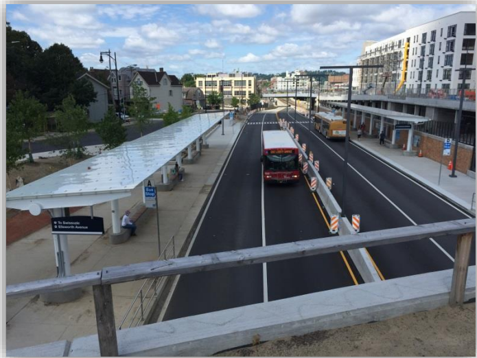
The East Busway serves 25,000 riders daily in a dense transit corridor. Possible expansion of the busway would reach suburban communities wanting improved transit service and help ease traffic congestion on commuter arteries.
