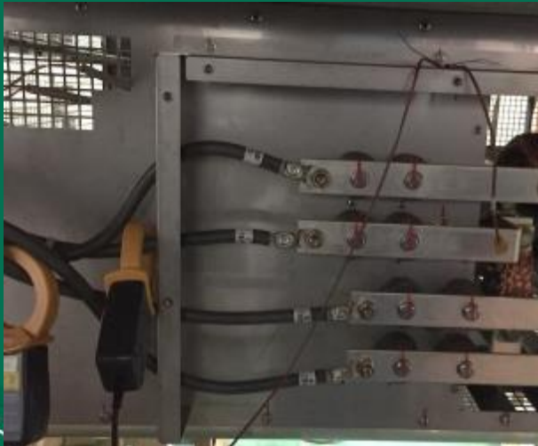
Swapping Polarity of BR connections
