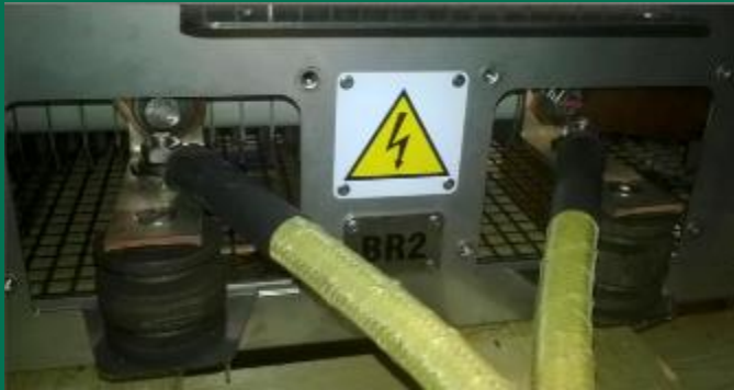
BR terminals and cable fanout
