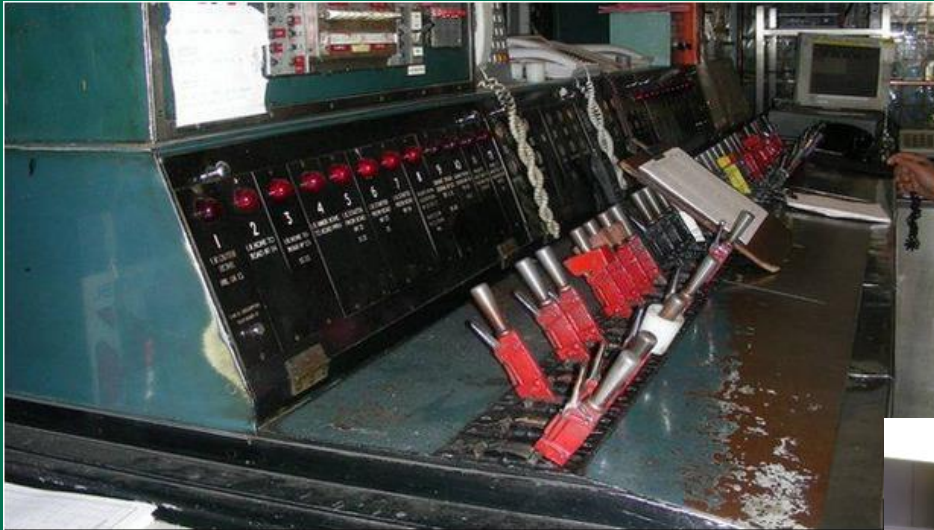
TfL said it needs to replace old signalling equipment
