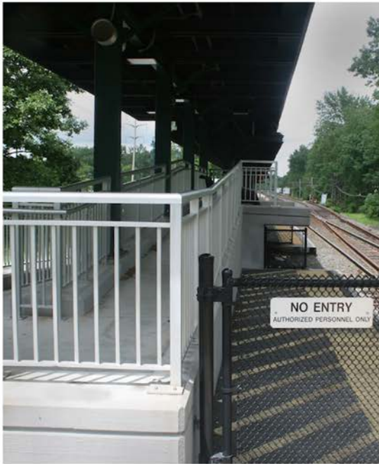
Mini-High Platform with Appropriate Barrier
