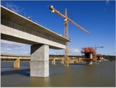
Construction & Bridge Building
