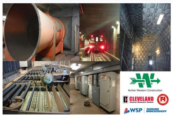
The Project will rehabilitate the TVS by inspecting, testing and then rehabilitating, replacing or upgrading individual components, assemblies and/or subsystems that make up the complete TVS with an overall program framework which minimizes risks to operations and safety.
