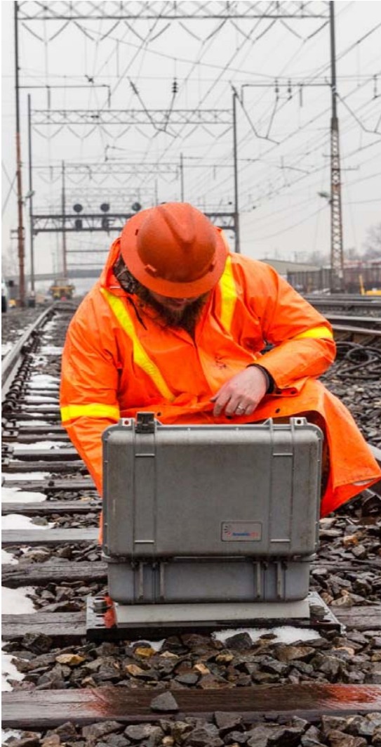
An Amtrak technician resetting a PTC transponder in Pennsylvania along the Northeast Corridor.
