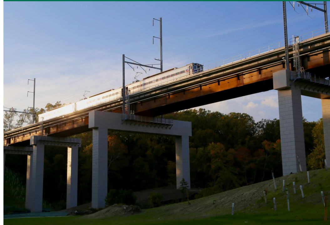
Completed Crum Creek Viaduct
