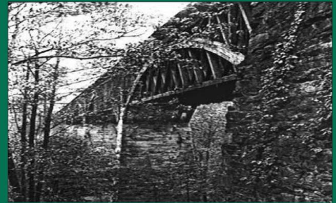
Wood and stone viaduct - constructed 1854
