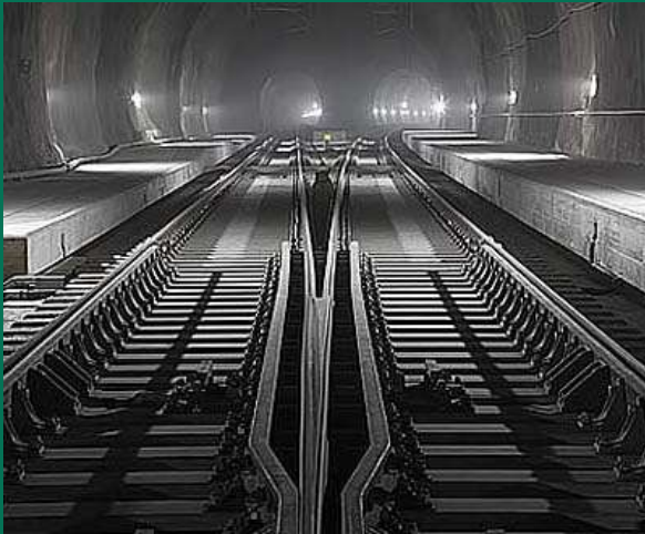
switch in the middle of the tunnel
