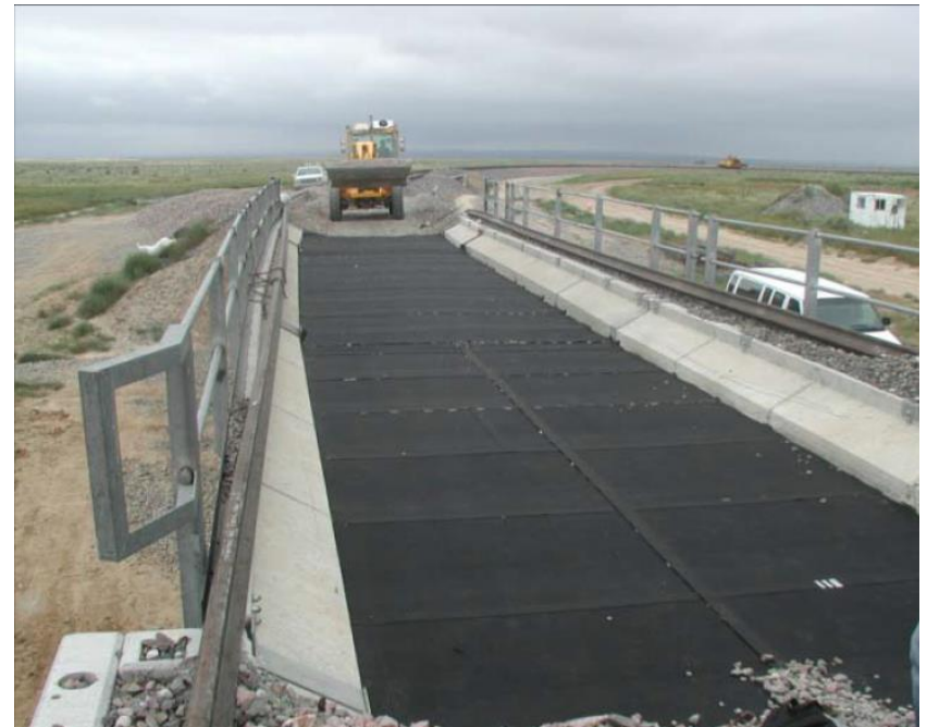
Mademann, C. and D. Otter. 2013. Effects Of Ballast Depth And Degradation On Stresses In Concrete Bridges . Transportation Technology Center, Inc.
