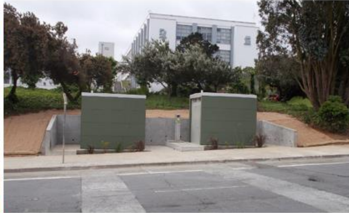
Geary Blvd. / 32nd Ave.
