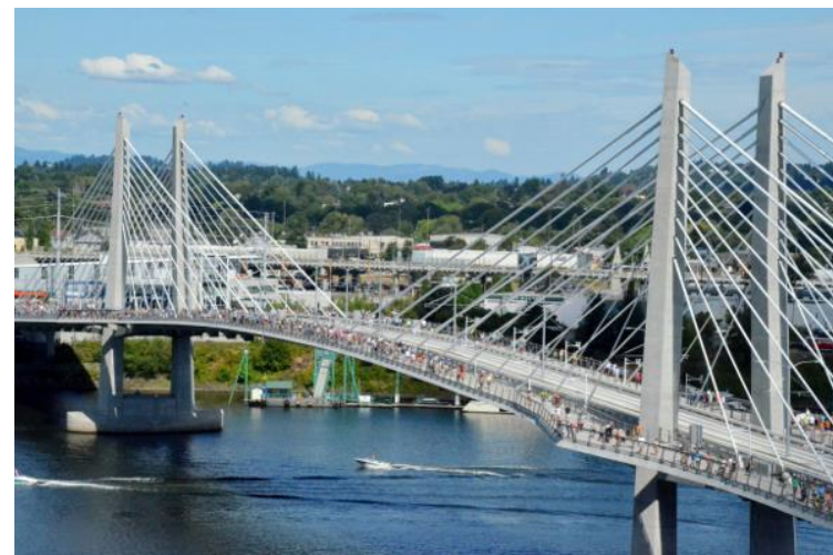
Willamette River Bridge, Portland
