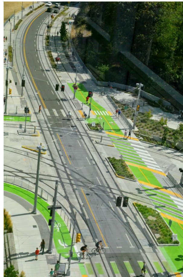
Southwest Moody Ave, Portland
