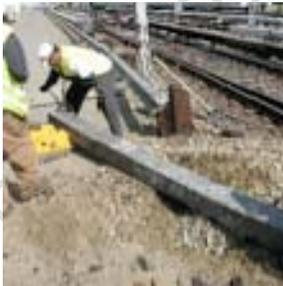
**Recycled Plastic Rail Ties: San Francisco Bay Area Rapid Transit (BART)** is swapping out worn wooden railroad ties with plastic ones made out of recycled grocery bags, milk bottles and old car tires. Plastic ties are stronger, lasting twice as long and are three times cleaner to make.
