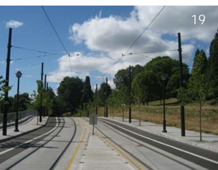
19: Streetcar simple overhead power supply supported by span wire; Portland, OR
