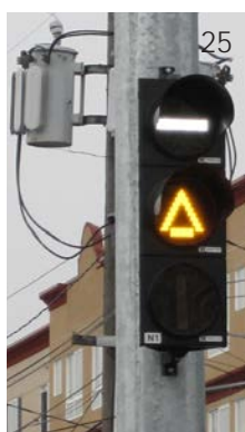
20: LRT grade crossing warning system; Charlotte, NC
