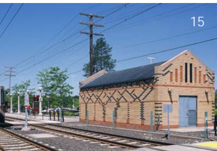
15: LRT substation with architectural treatment; Portland, OR
