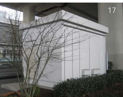
17: Streetcar substation factory-assembled; Portland, OR
