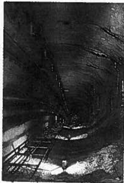
A Port Authority of Allegheny County light rail tunnel in Pittsburgh with walls left in a natural state. Some tunnels have finished walls and several tracks.
