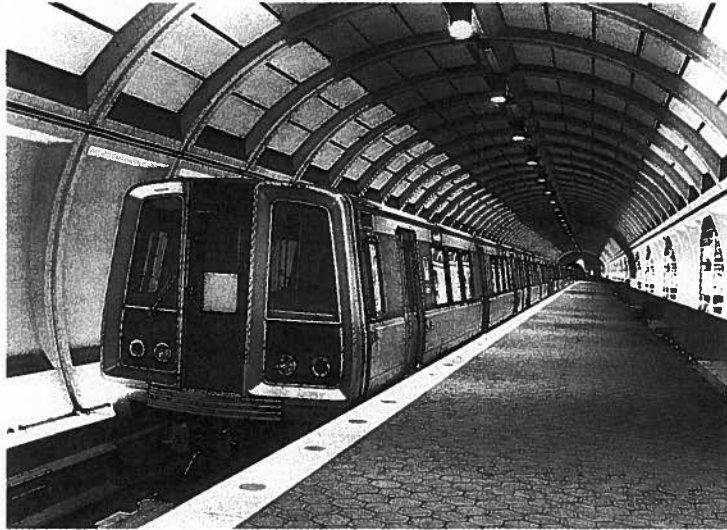
Modern rail station design minimizes crime by eliminating columns, dark corners, and other areas where criminals can lurk. This Washington Metropolitan Area Transit Authority heavy rail station illustrates such design.
