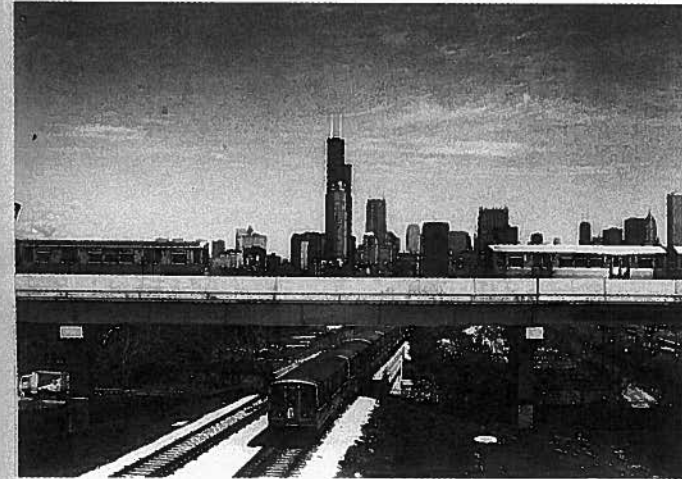
The Chicago Transit Authority operates all three types of rail fixed guideway--surface and elevated, shown here, and tunnel.
