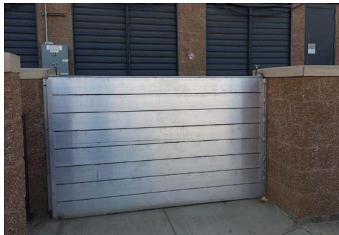
Permanent flood wall with deployable shield
