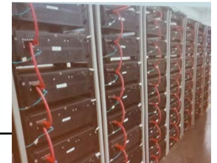
Smart Microgrid + Second Life Li-Ion Energy Storage
