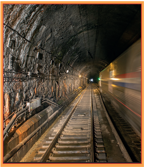
An Amtrak train passing through the current B&P tunnel.
