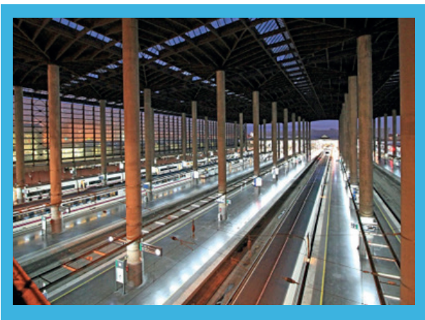
Figure 3: Madrid Atocha HSR Station.
