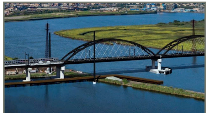
ABOVE: THE NEW PORTAL NORTH BRIDGE WILL RISE MORE THAN 50 FEET OVER THE HACKENSACK RIVER, NEGATING THE NEED TO OPEN AND CLOSE FOR RIVER TRAFFIC.
