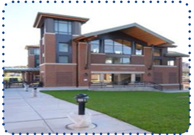
MERIDEN STATION, ONE OF THREE NEW STATIONS ON THE HARTFORD LINE
