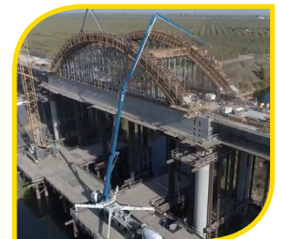
California High-Speed Rail San Joaquin River Viaduct under construction in 2020.
