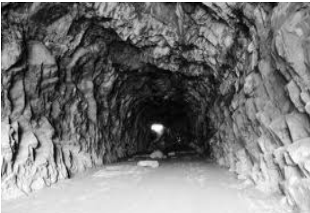
Unlined Rock Tunnel
